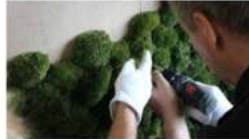
2 Utilise the help of another person during the installation; this allows one person to press the panels firmly against the wall while the other screws them tight. Image: Freund GmbH
