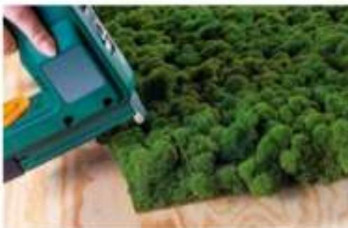
The moss panels can be either stapled, screwed or directly glued to a wooden subsurface.
