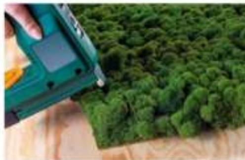
The moss panels can be either stapled, screwed or directly glued to a wooden subsurface.
