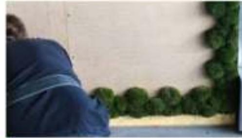
1 Always start the installation at the bottom (if needed with the help of a wooden strip) and work your way up. Image: Freund GmbH
