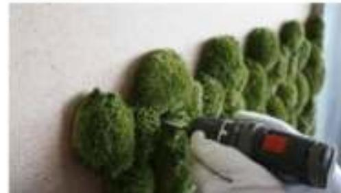
3 Ideally, the installation is carried out on a carrier panel. Keep an eye out for small gaps in the moss for placing the screws during the installation of our product. Image: Freund GmbH
